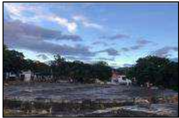
Tanque San Luis No.1
