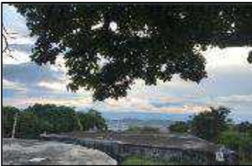
Tanque San Luis No.2
