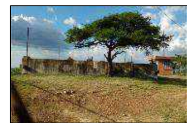
Tanque Santo Domingo
